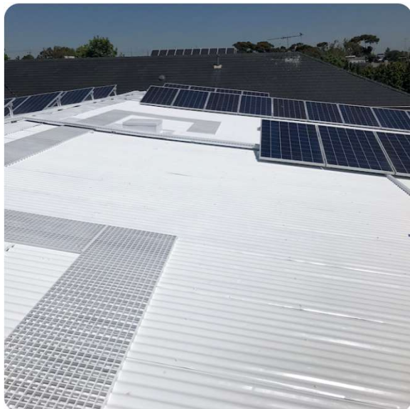
Photo of 'cool roof' painting on Bradshaw Street Community Hall, Essendon
